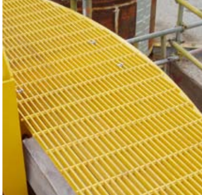
Gratings for platform Pultruded gratings serves as platforms in oil refineries.
