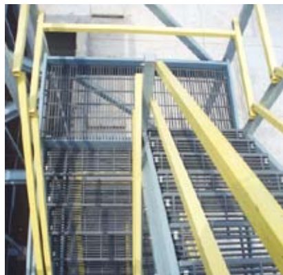
Stair Tread Stair tread installed on offshore access ramps withstand corrosion, wear and tear.
